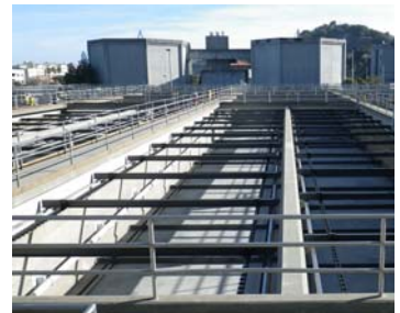
Launders after sandblasting (left) and Primary Clarifier No. 2 with new coating
