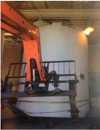
New tank being carefully positioned.
