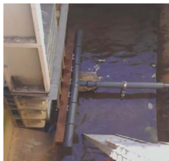
...and ready for testing.
