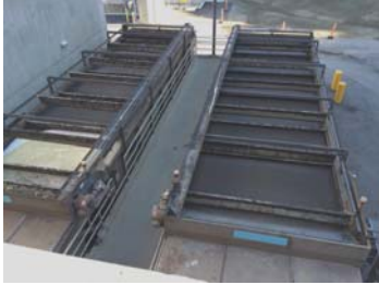
DAF thickeners to be replaced.
