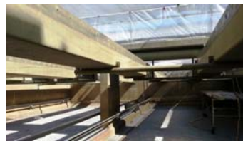
Launders after sandblasting (left) and Primary Clarifier No. 2 with new coating
