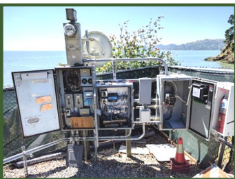
Patchwork of control panels assembled over five decades.
