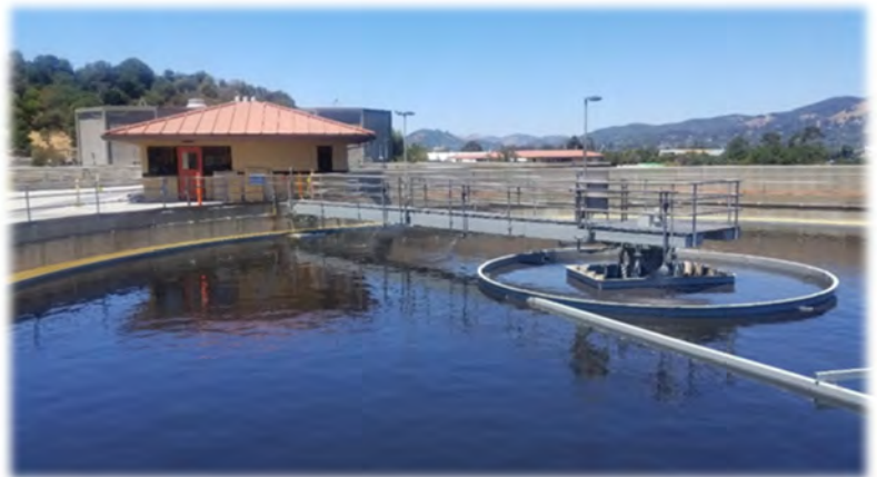
Secondary Clarifier No. 3 in service after rehabilitation.
