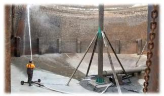
removed in August, and the sludge, struvite, and grit that had accumulated inside the digester were removed in September. Staff is taking advantage of the shutdown to inspect the tank and perform preventative maintenance work on the digester valves and piping before the new membrane cover is installed in October. Digester No. 2 is expected to return to service in early November.
