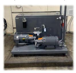
operators for the Primary Clarifiers were replaced with electric operators. Due to the unit being 37 years old and now oversized, it was replaced with a skid mounted and self-contained unit equipped with two motors and pumps, fluid storage tank, and a control panel. Mechanical technicians installed the new unit and Electrical/ Instrumentation technicians connected it to the SCADA system and an emergency use only portable generator transfer switch.
