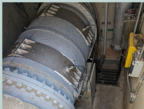
Proposed new flowmeter for the Ross Valley Interceptor
