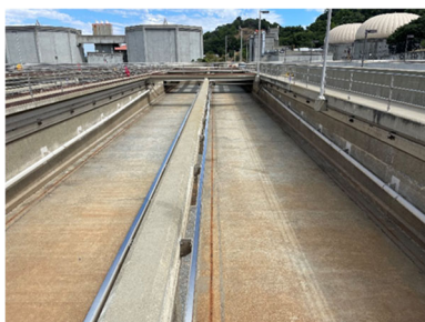
Primary Clarifier No.1 being rehabilitated in 2024
