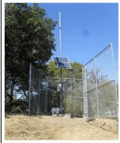
In July, our selected location for the repeater station was approved by San Rafael's Planning Department, the repeater base was set in place with concrete, and Coggins Fencing installed a no climb fence. This month CMSA staff fastened the repeater radio to its base, installed the control panel, and mounted a solar powered electrical source. A master radio and antenna mounted on top of the CMSA Administration Building will transmit and receive pump station information in the near future.
