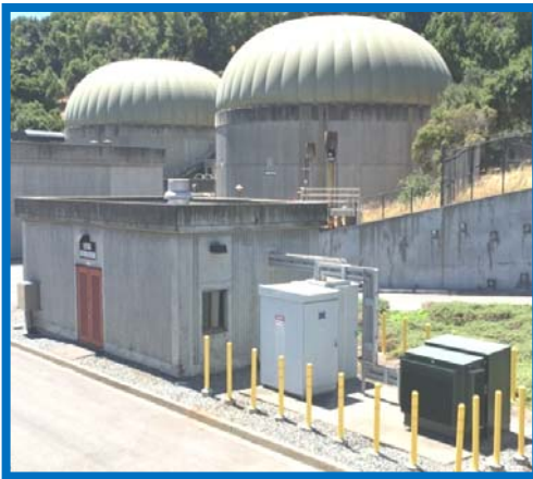
PG&E transformer and main plant switchgear; cogeneration engine.
