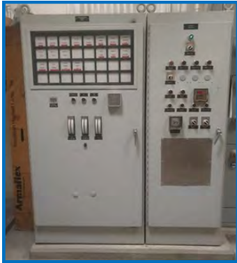
Existing control cabinet at SQPS needing replacement.
