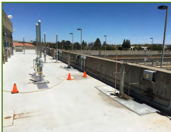
Existing hydraulically-operated primary clarifier gate systems.
