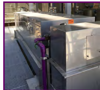
Rotary drum thickeners, one of the many Agency assets.
