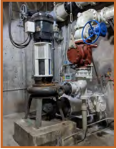
Direct-coupled pump with enclosed rotating equipment.
