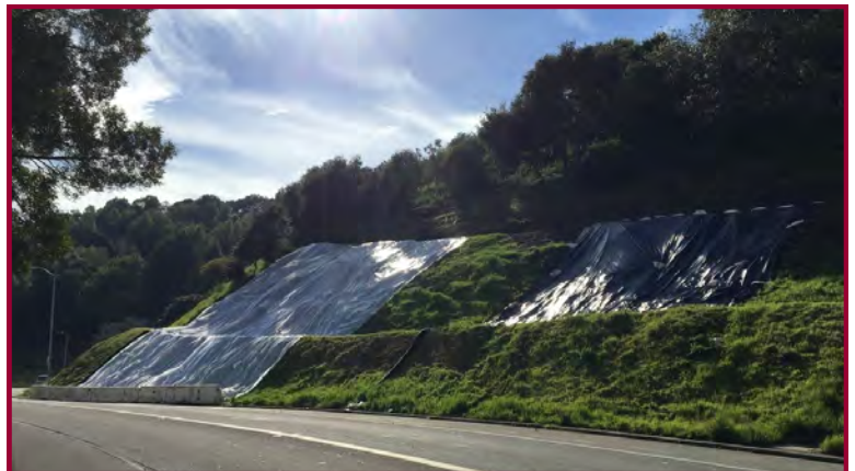
Landslide sites on Andersen Drive with tarps for temporary protection.
