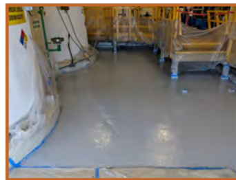
New coating in bisulfite storage room, spalled concrete in hypochlorite vault.
