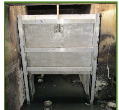
New isolation gate in place.
