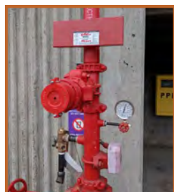
Fire protection water riser with new spare head box and drain valve.
