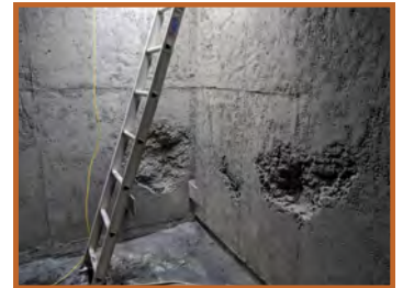
New coating in bisulfite storage room, spalled concrete in hypochlorite vault.
