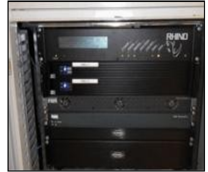
Pictured, the new VoIP system
