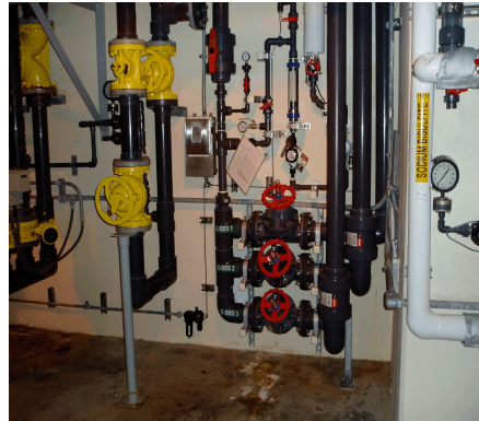
Emergency De-Chlorination System Supply Header
