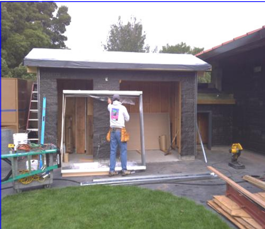
Pictured above: A contractor is getting ready to install the door frame at the public education materials storage shed.
