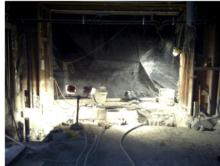
Demolition of former ladies locker room
