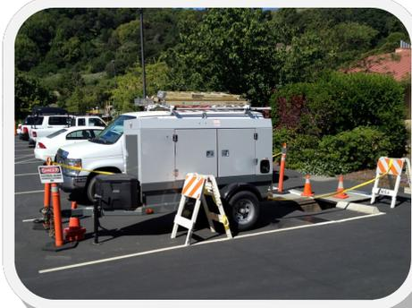
Staff has successfully performed four plant shutdowns this year with one more scheduled for the immediate future. The procedure involves temporarily unplugging CMSA from PG&E, shutting-down our Cogeneration system, and using a portable generator (left) to power the Administration building. Treated water is diverted to offline tanks and the storage pond during the shutdowns while contractors and staff perform electrical upgrades for the Digester Project.
